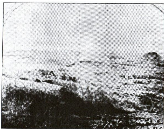
Detail of the Greensward #5, Photograph of area of park before construction, 1858.
