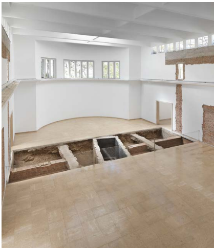
10 Maria Eichhorn, Relocating a Structure . German Pavilion 2022, 59th International Art Exhibition – La Biennale di Venezia, 2022, detail: Joins between sections of the building from 1909 and 1938; doorway to the left rear side room from 1909, walled up in 1928; foundations of the rear wall from 1909; rear wall of the building from 1909; interior wall from 1938, demolished in 1964; wall lettering; doorway to the right side room from 1909, walled up in 1912, exhibition view, © Maria Eichhorn / VG Bild-Kunst, Bonn 2022, photo: Jens Ziehe
