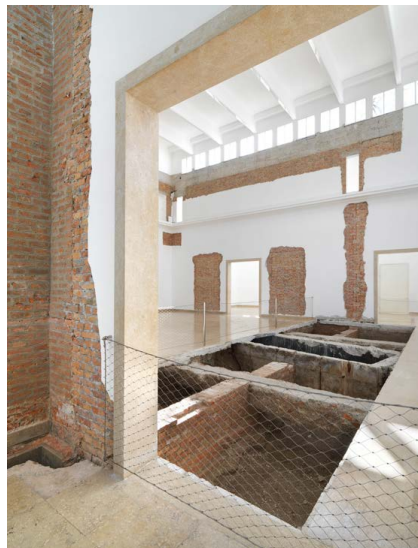
5 Maria Eichhorn, Relocating a Structure . German Pavilion 2022, 59th International Art Exhibition – La Biennale di Venezia, 2022, detail: Rear wall of the building from 1909, plastered as an interior wall in 1938; join between sections of the building from 1909 and 1938; wall lettering; doorway to the left front side room from 1909, walled up in 1938; doorway to the left rear side room from 1909, walled up in 1928; rear wall of the building from 1909, interior wall from 1938, demolished in 1964; foundations of the rear wall from 1909, exhibition view, © Maria Eichhorn / VG Bild-Kunst, Bonn 2022, photo: Jens Ziehe
