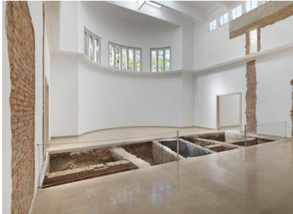
7 Maria Eichhorn, Relocating a Structure . German Pavilion 2022, 59th International Art Exhibition – La Biennale di Venezia, 2022, detail: Doorway to the left rear side room from 1909, walled up in 1928; foundations of the rear wall from 1909; join between sections of the building from 1909 and 1938; rear wall of the building from 1909; interior wall from 1938, demolished in 1964; wall lettering; doorway to the right side room from 1909, walled up in 1912, exhibition view, © Maria Eichhorn / VG Bild-Kunst, Bonn 2022, photo: Jens Ziehe
