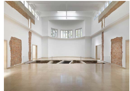
9 Maria Eichhorn, Relocating a Structure . German Pavilion 2022, 59th International Art Exhibition – La Biennale di Venezia, 2022, detail: Joins between sections of the building from 1909 and 1938; wall lettering; doorway to the left rear side room from 1909, walled up in 1928; foundations of the rear wall from 1909; rear wall of the building from 1909; interior wall from 1938, demolished in 1964; doorway to the right side room from 1909, walled up in 1912, exhibition view, © Maria Eichhorn / VG Bild-Kunst, Bonn 2022, photo: Jens Ziehe
