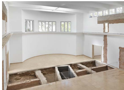
11 Maria Eichhorn, Relocating a Structure . German Pavilion 2022, 59th International Art Exhibition – La Biennale di Venezia, 2022, detail: Joins between sections of the building from 1909 and 1938; doorway to the left rear side room from 1909, walled up in 1928; foundations of the rear wall from 1909; rear wall of the building from 1909, interior wall from 1938, demolished in 1964; wall lettering; doorway to the right side room from 1909, walled up in 1912, exhibition view, © Maria Eichhorn / VG Bild-Kunst, Bonn 2022, photo: Jens Ziehe
