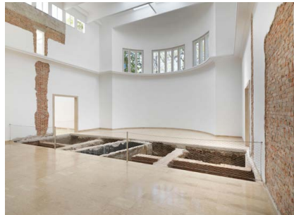
8 Maria Eichhorn, Relocating a Structure . German Pavilion 2022, 59th International Art Exhibition – La Biennale di Venezia, 2022, detail: Join between sections of the building from 1909 and 1938; foundations of the rear wall from 1909; rear wall of the building from 1909, interior wall from 1938, demolished in 1964; doorway to the right side room from 1909, walled up in 1912, exhibition view, © Maria Eichhorn / VG Bild-Kunst, Bonn 2022, photo: Jens Ziehe
