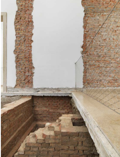
1 Maria Eichhorn, Relocating a Structure . German Pavilion 2022, 59th International Art Exhibition – La Biennale di Venezia, 2022, detail: Foundations of the rear wall from 1909; rear wall of the building from 1909, interior wall from 1938, demolished in 1964; wall lettering; chimney from an earlier building (undated); doorway to the right side room from 1909, walled up in 1912, exhibition view, © Maria Eichhorn / VG Bild-Kunst, Bonn 2022, photo: Jens Ziehe
