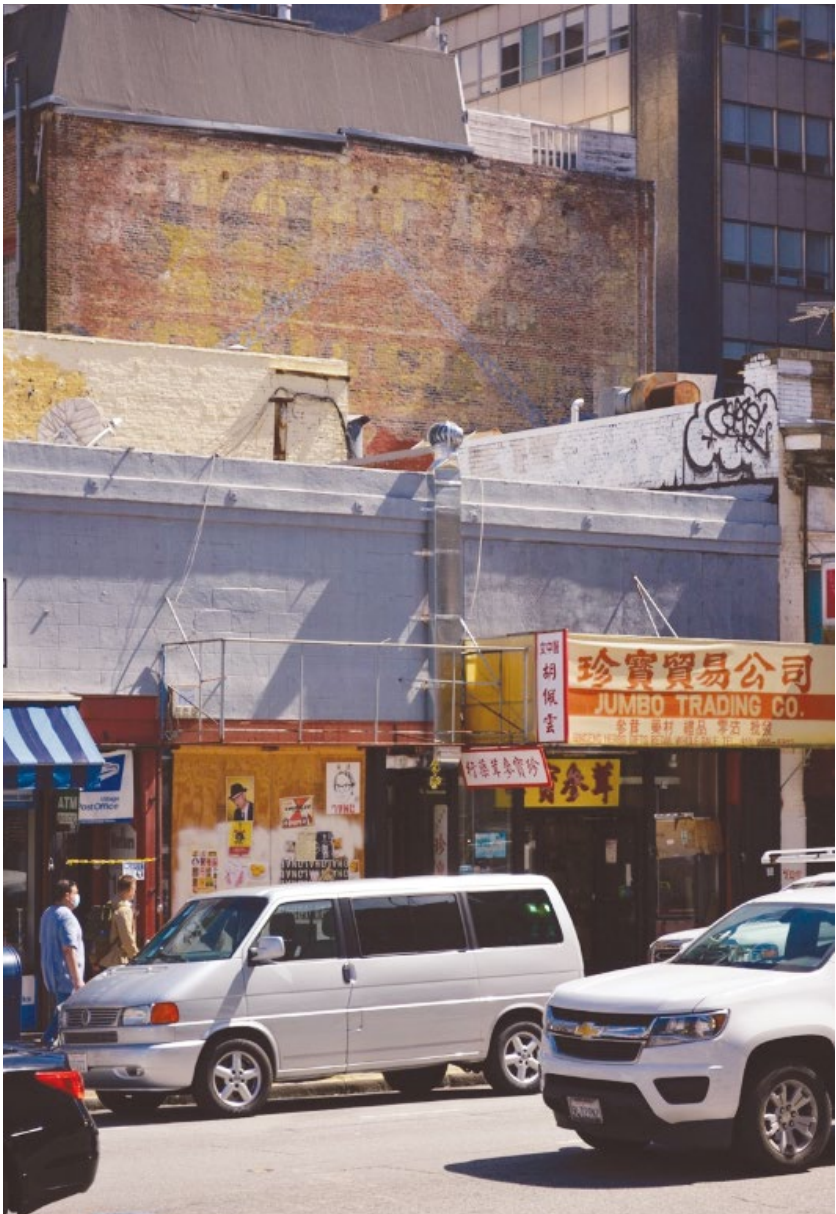
Installation of ductwork and whirlybird turbine ventilator on the exterior of Pied-à-terre, San Francisco, 2022. Photography by McIntyre Parker.
