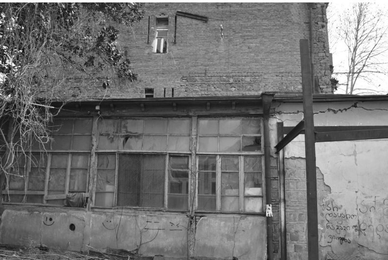
Former tenement house at 49 Tsinamdzgvrishvili Street. Tbilisi. Side elevation.
