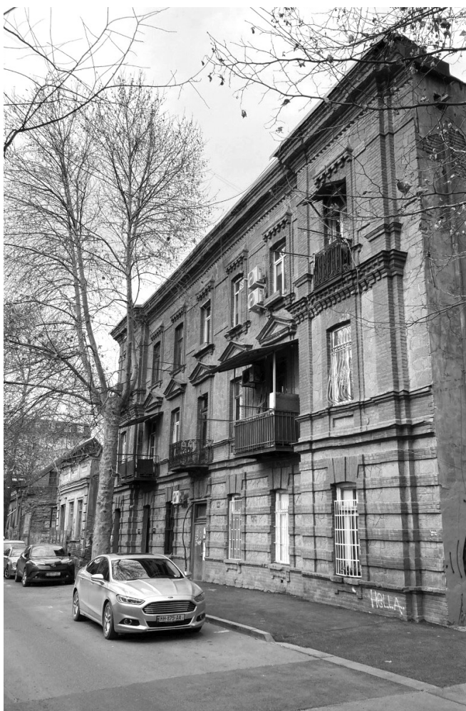
Former tenement house at 49 Tsinamdzgvrishvili Street. Tbilisi. Main façade. 5
