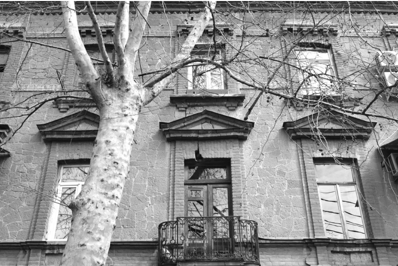
Former tenement house at 49 Tsinamdzgvrishvili Street. Tbilisi. Fragment of main façade.
