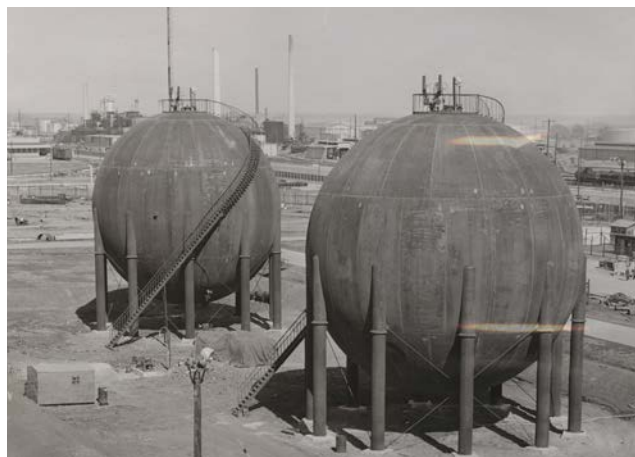
Clémence de La Tour du Pin. TPC Group [Modifications and Additions to Process Facilities], 1953. Historical photograph on loan from Special Collections UH Libraries, 8 x 10 in. Courtesy of the artist.
