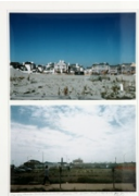
Top: New 'Monster' Houses under Construction , Vancouver, 1999
